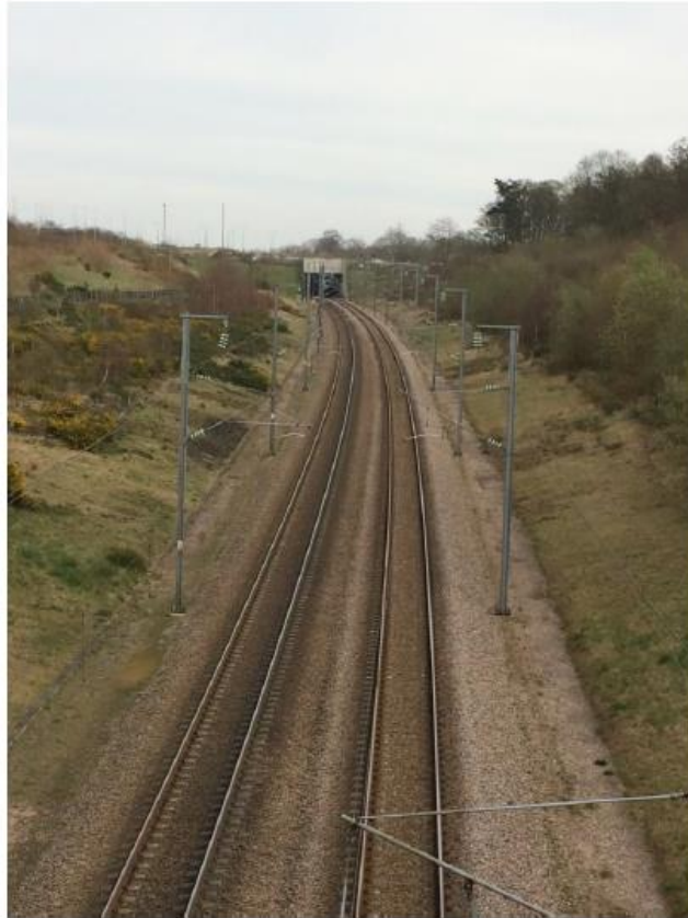
Approach to Medway Viaduct
